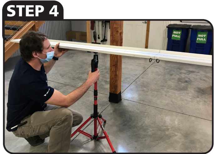
USE THE PRECISION PUMP JACK TO LEVEL FENCES
